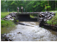
Road crossings that can withstand flood events (USFS, Monongahela NF)
