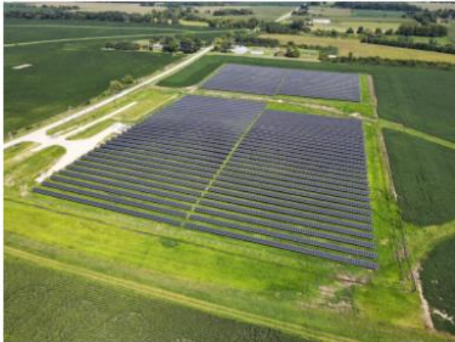
An Illinois Nexamp project currently in operation (Source: PRNewswire)
