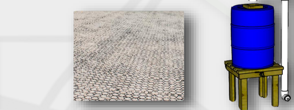
Left: Rain gardens collect water runoff and provide the time necessary for it to be absorbed into the ground. Center: Permeable pavement can be used for walkways or parking lots to prevent runoff. Right: Simple water catchment system, such as this rain barrel, can provide water throughout the growing season to water gardens and plants.
