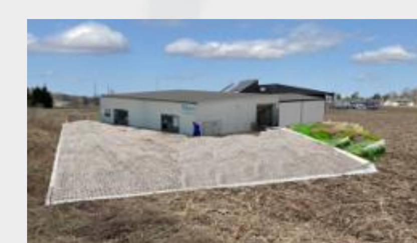
Green infrastructure, such as pervious pavements and rain gardens implemented at an aquaponics facility.
