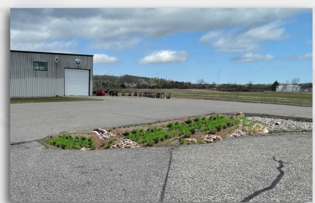
Left: Rain gardens collect water runoff and provide the time necessary for it to be absorbed into the ground. Center: Permeable pavement can be used for walkways or parking lots to prevent runoff. Right: Simple water catchment system, such as this rain barrel, can provide water throughout the growing season to water gardens and plants.
