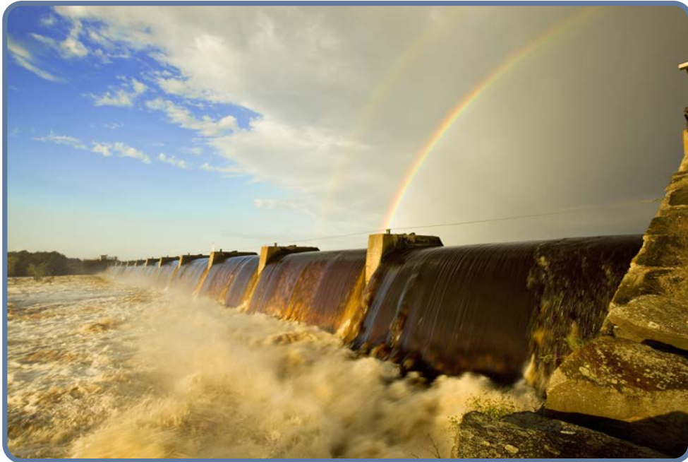
Spillways at Wissota Hydro. Located on the Lower Chippewa River, this facility was completed in 1918 and produces 36.4 MW. Photo Courtesy of Xcel Energy.
