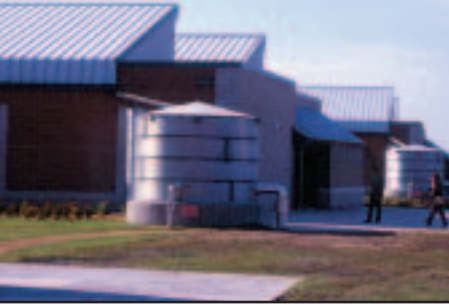
Roy Lee Walker Elementary School, in McKinney, TX, collects 700,000 gallons of rainwater each year.
