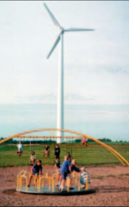
Photo: American Wind Energy Association The wind turbine at Spirit Lake Elementary, in Spirit Lake, IA, saves the school $25,000 annually.
