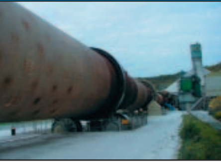
Photo: BuildingGreen Inc.
