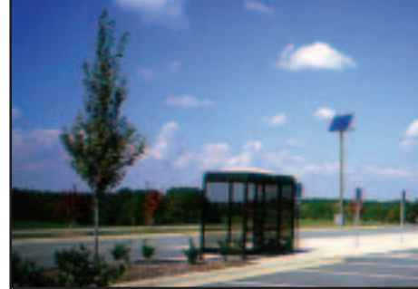
These stand-alone photovoltaic systems power parking lights.
